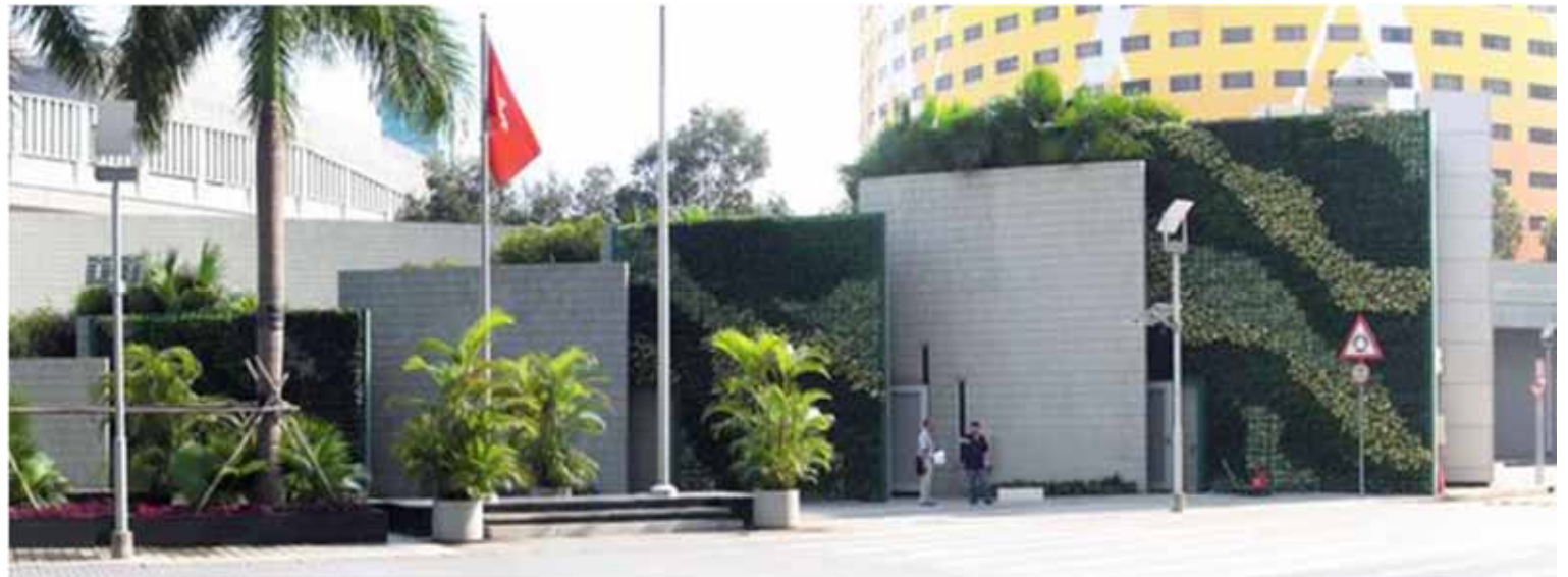
For a government building (EMSD Headquarters)
