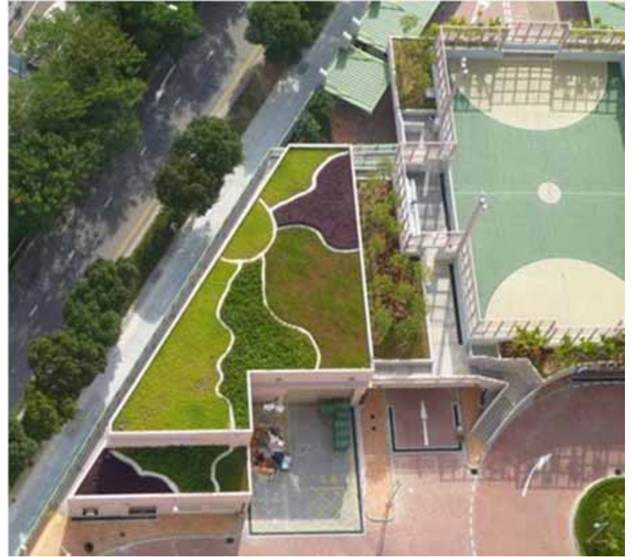
Refuge room 垃圾房
