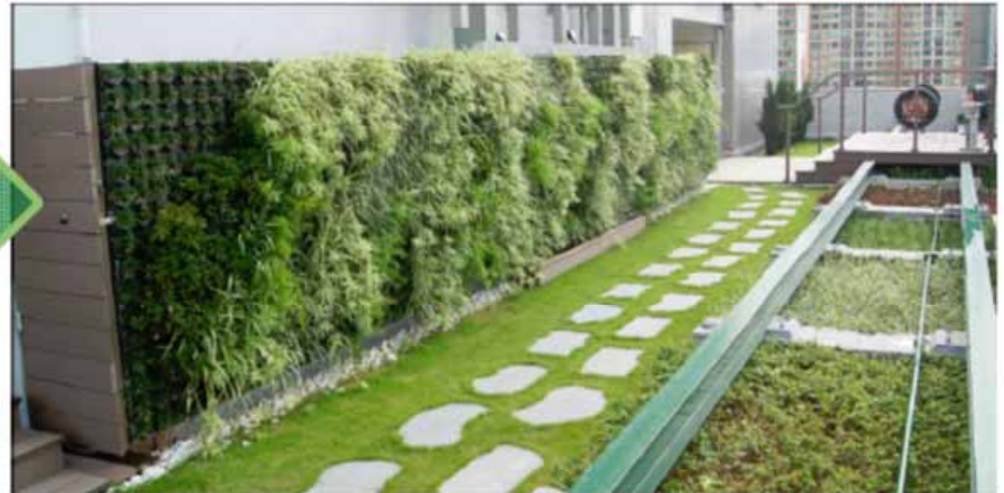
Paving and vertical greening on roof garden
