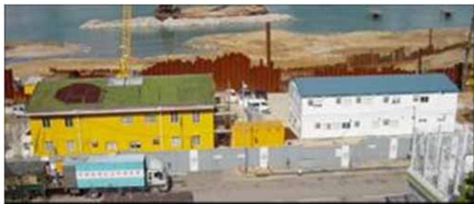
Green site office and typical site office
