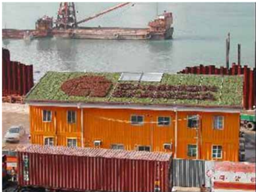
Green site office
