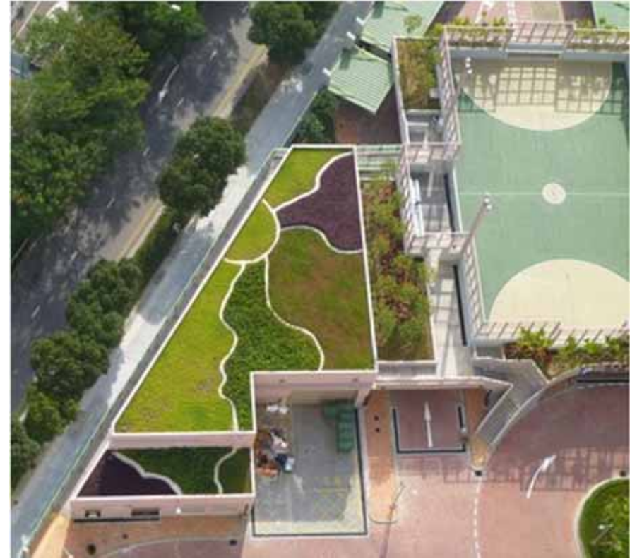
Refuge room 垃圾房
