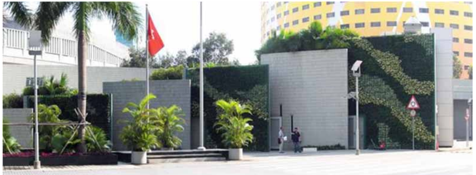
For a government building (EMSD Headquarters)
