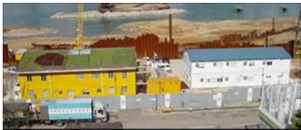
Green site office and typical site office
