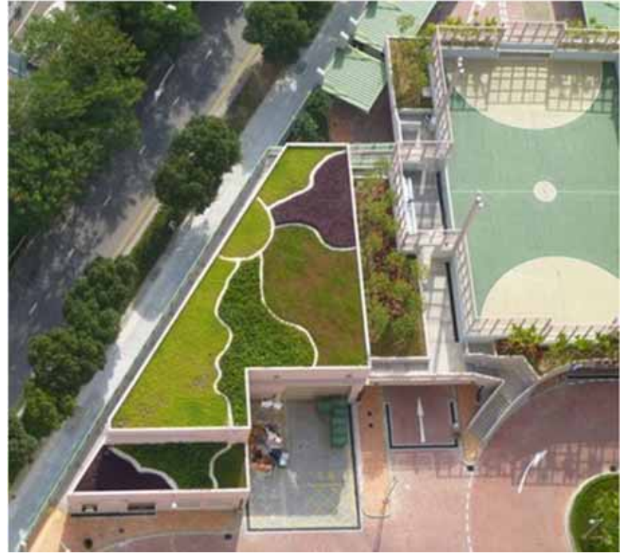
Refuge room 垃圾房
