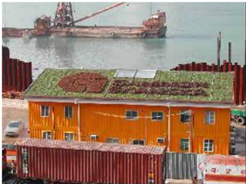
Green site office
