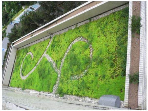
1/F green roof (13 Aug 2009)
