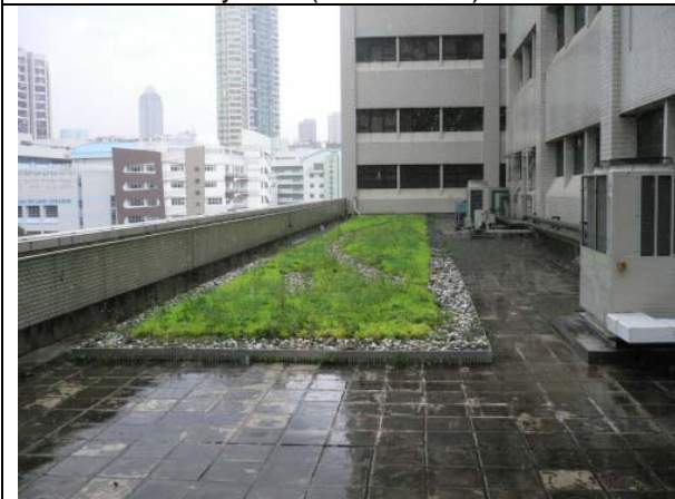
4/F green roof (6 Aug 2009) (rainy day)
