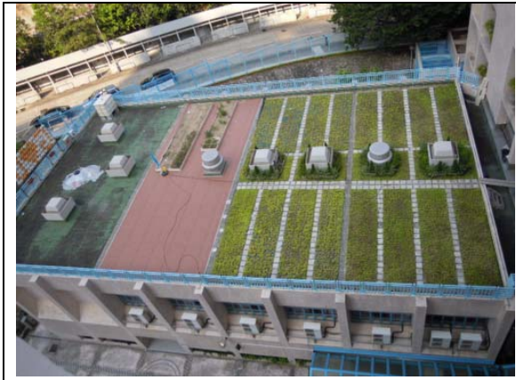
Overview of assembly hall (5 Sep 2009)
