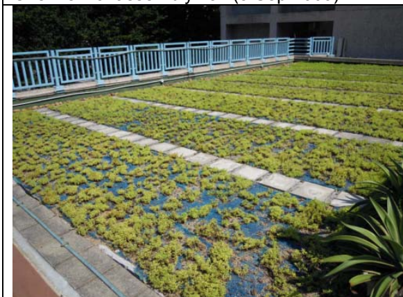
Extensive green roof (5 Sep 2009)
