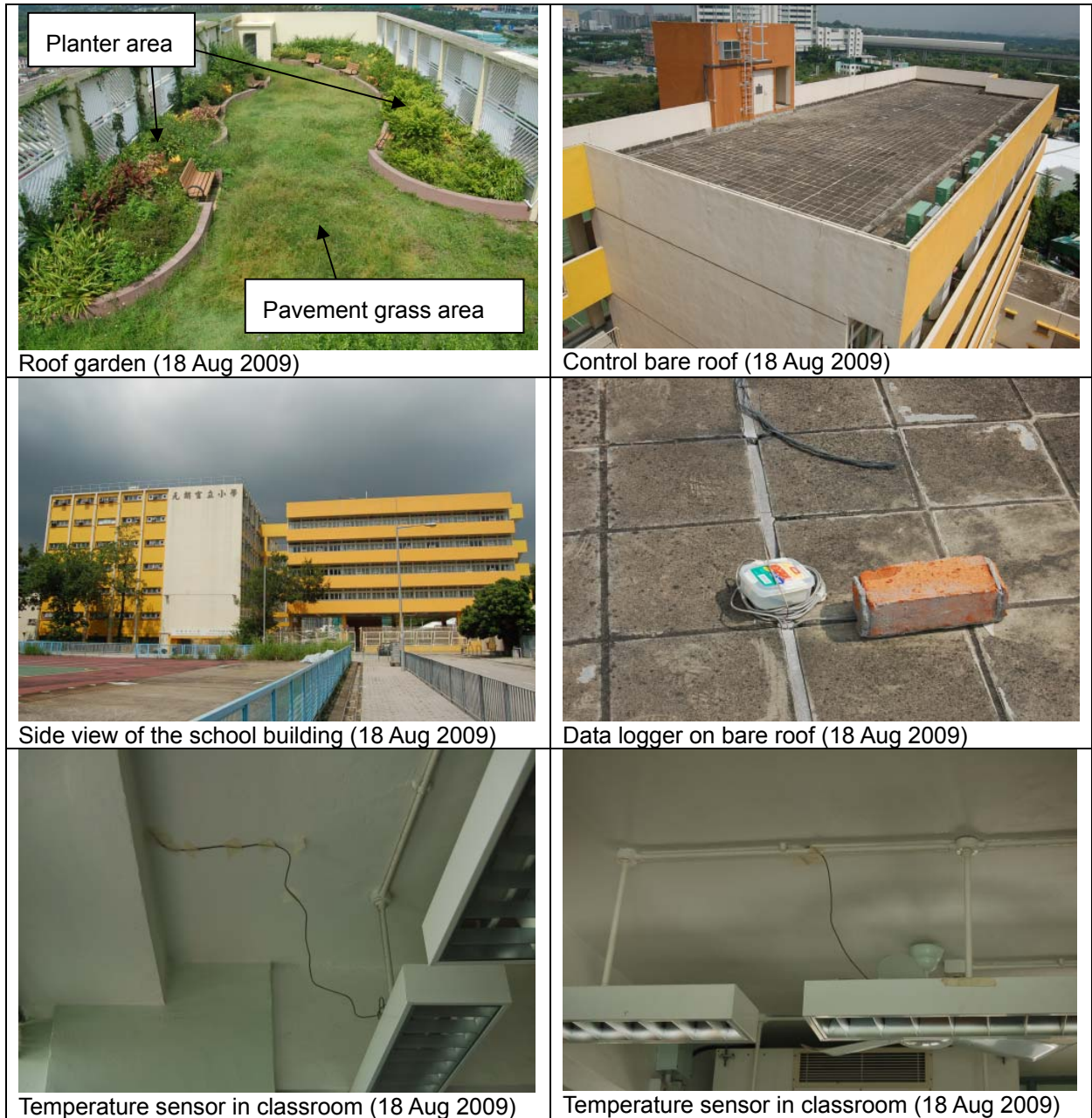
Figure A7.2 Selected site photos of YLGPS
