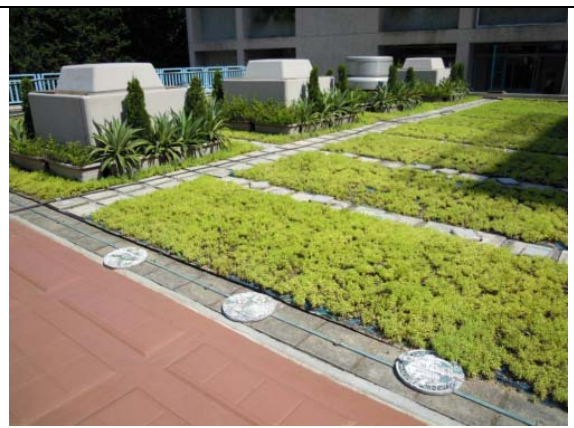
Extensive green roof (5 Sep 2009)
