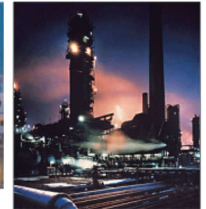
Petrochemical plant lighting
