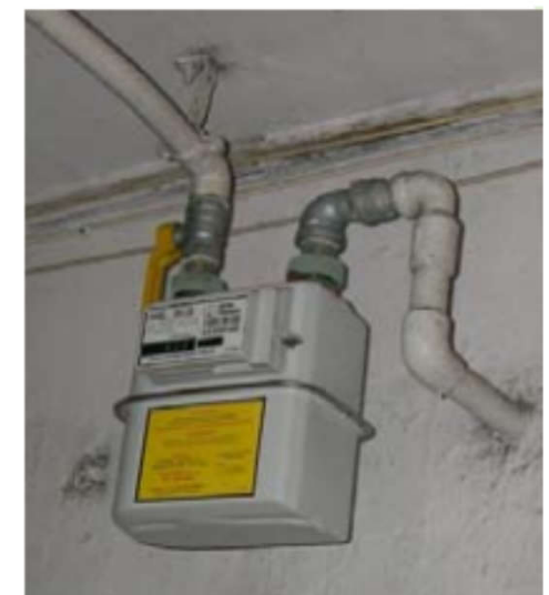
Figure 3: An installation pipe and gas fittings
