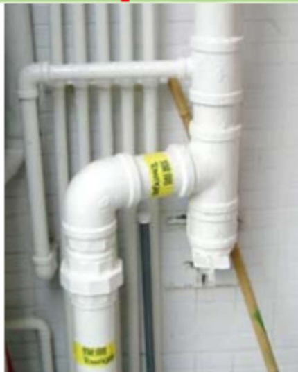
Figure 1: Vertical sections of a service riser
