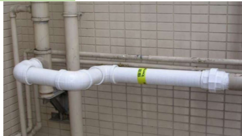
Figure 2: Horizontal sections of a service riser
