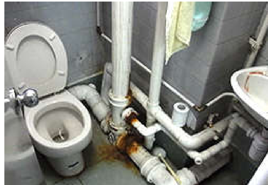
Rusty internal drainage pipes
