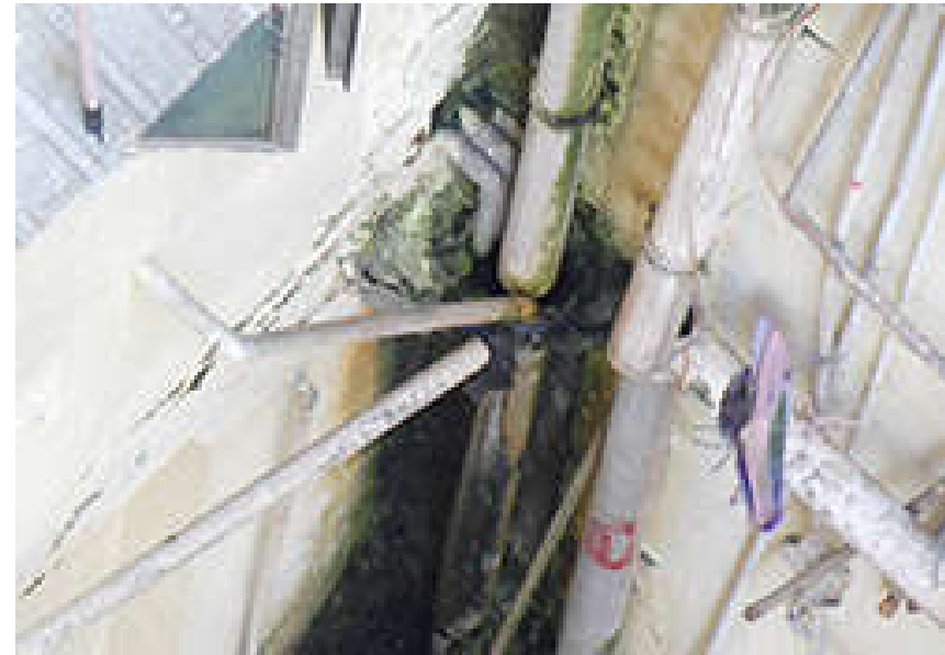
Unauthorised alteration of drainage system
