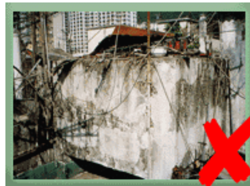
Storage tank without proper maintenance & management
