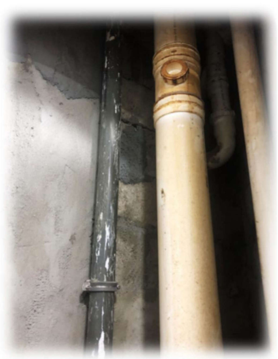
Internal pipe duct accessible from common parts
