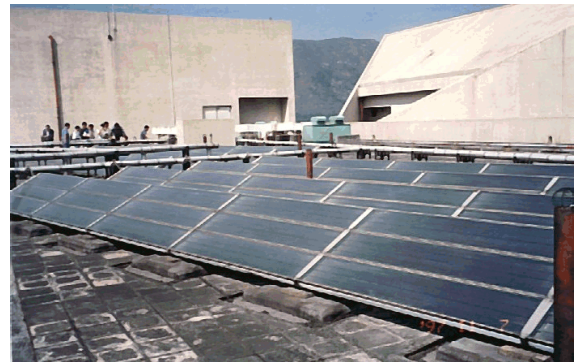
Solar hot water system in a hospital in Tuen Mun
