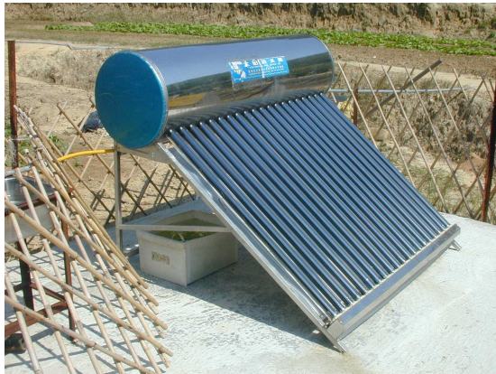
Evacuated-tube solar hot water system
