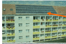
Solar collectors integrated with roof
