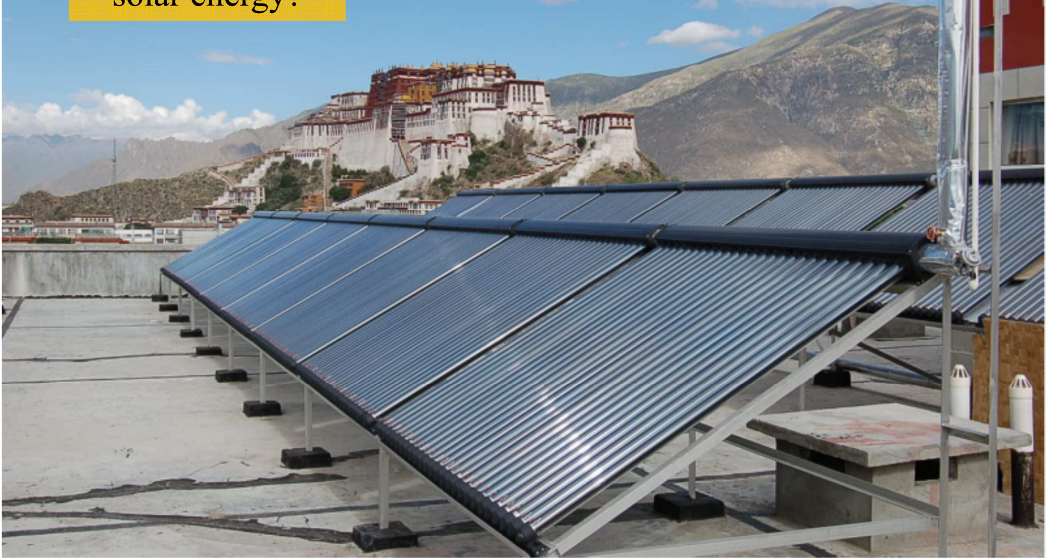
Evacuated-tube solar hot water system in a hotel in Lhasa, Tibet (photo taken by Dr Sam C M Hui)
