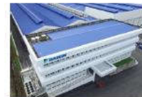
Daikin Chiller & AHU Manufacturer AC Split unit Manufacturer
