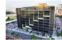
Pam Building Green Building
