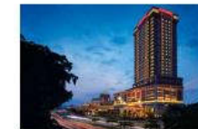
Sunway Clio Hotel Intrix Hot Water System
