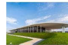
Setia City Convention Center Green Building
