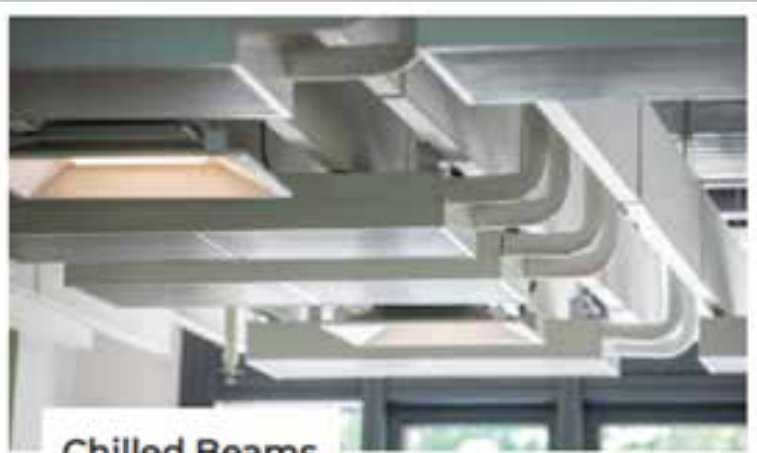
Chilled Beams
