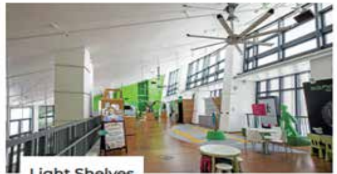
Light shelves on its southeast and northwest facades shade the periphery and distribute daylight furthest away from the windows
